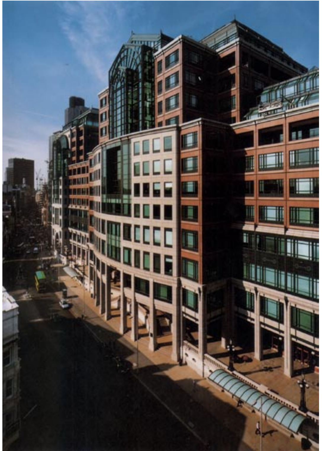
Broadgate's 135 & 155 Bishopsgate blocks are 'PLATTENBAU BEAUX ARTS' - East Germany's answer to Paris. They are built of panels, one storey high and one window wide. Check the black lines. The walls are thin slices of granite glued to a light steel frame. The openings are a big sheet of plate glass decorated by stuck-on 'Chicago' window-bars.
